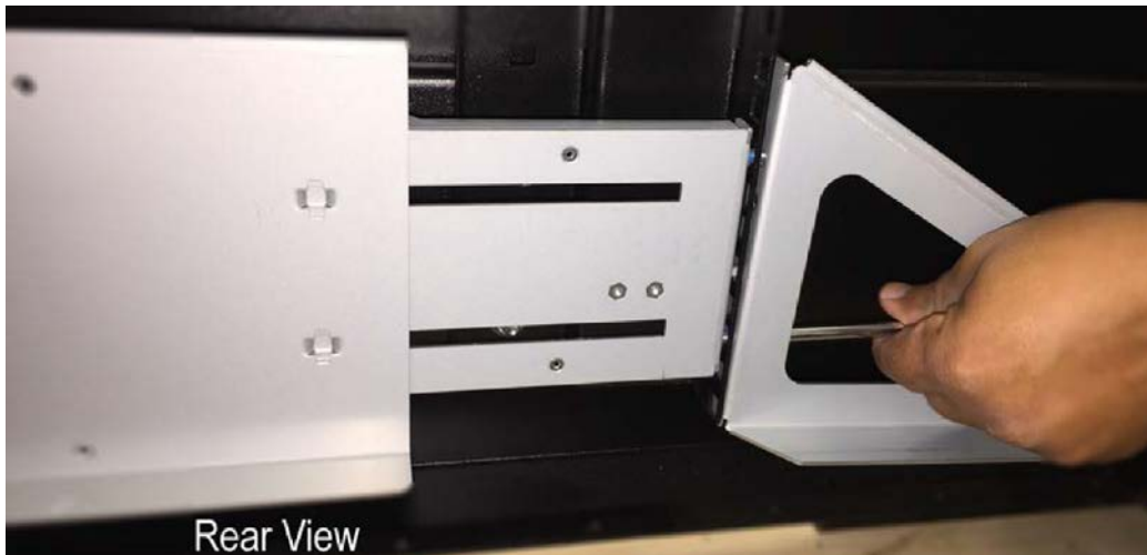
Figure 3-97. Back End to Rear Vertical Rail
