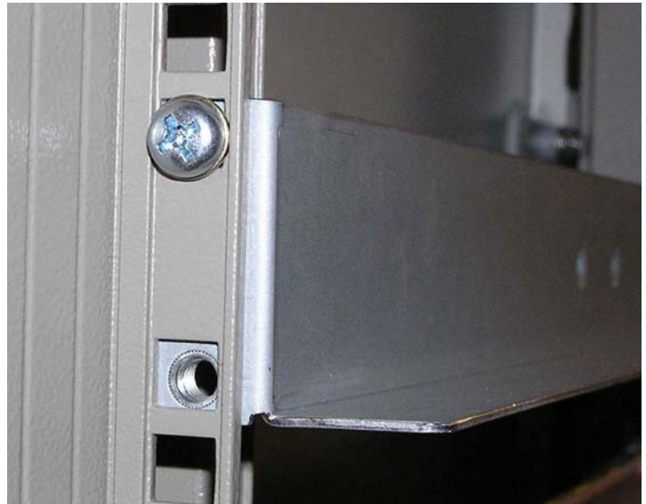
Figure 3.4 Rack mounting kit mounted in rack
